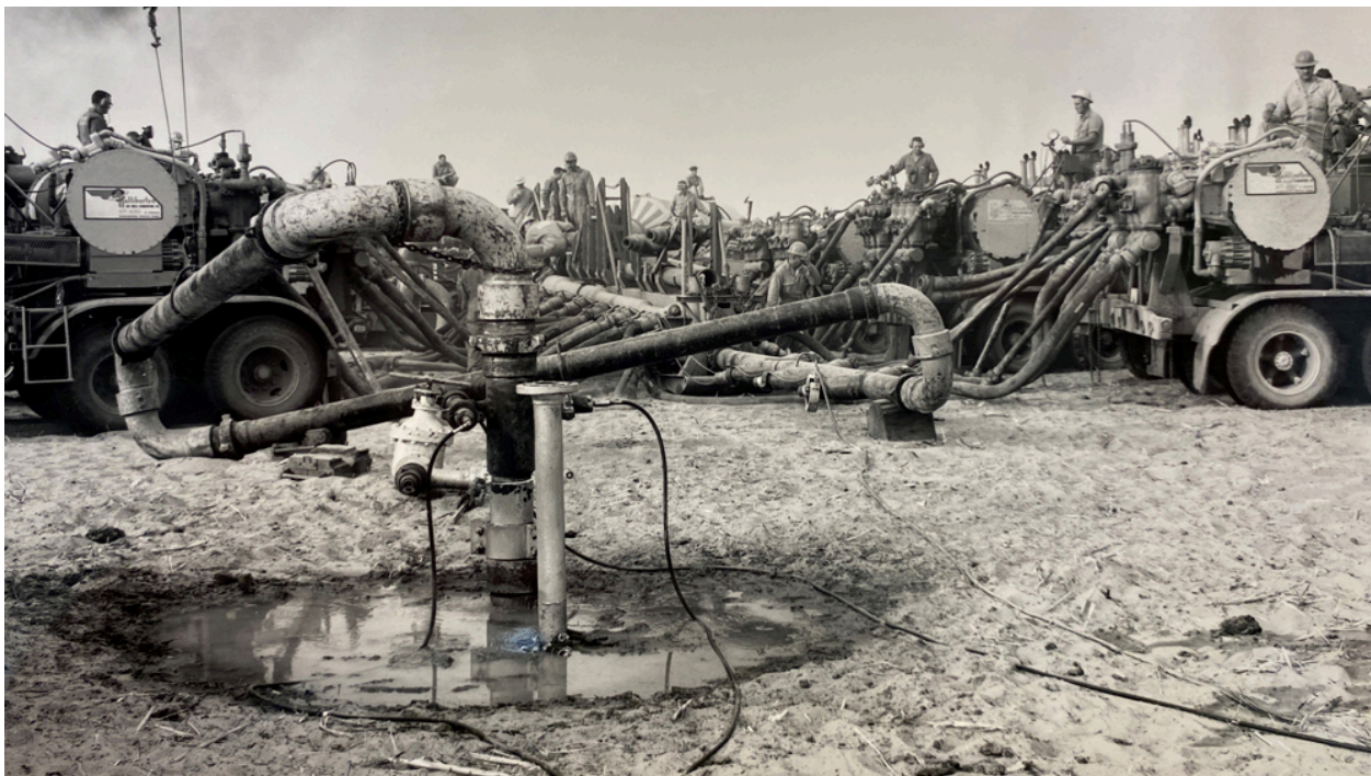
Fig. 3. By 1963, multi-pump spreads added horsepower, but every decision was still made manually.
