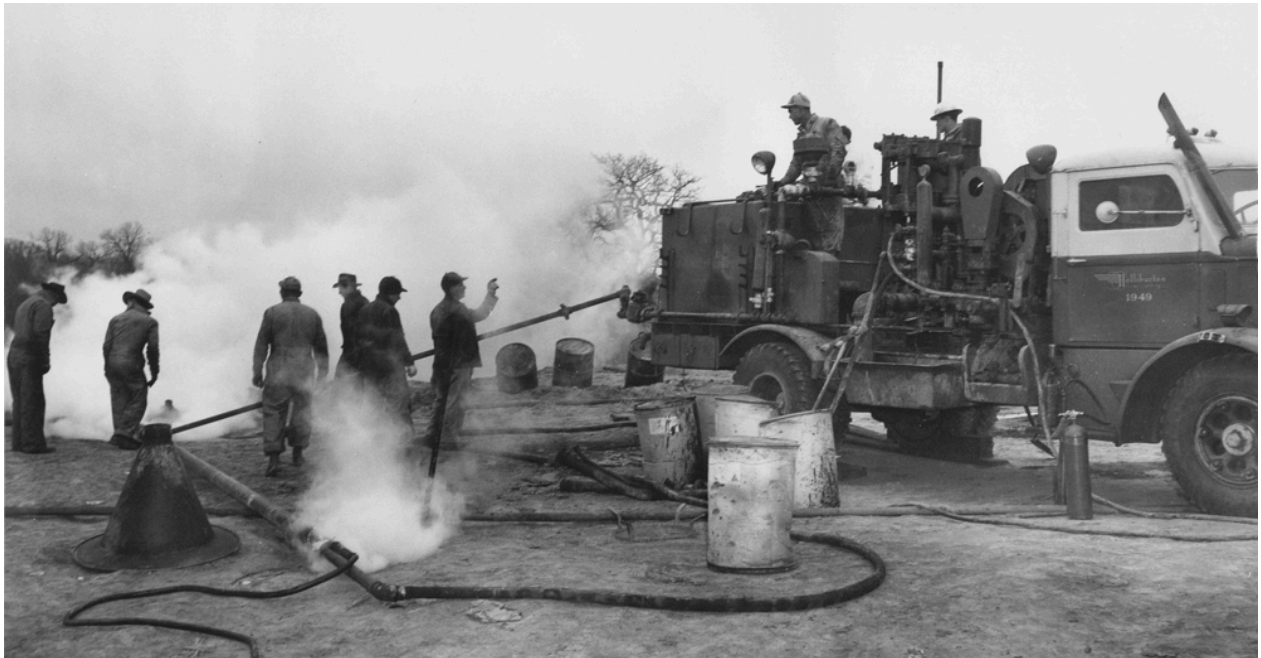
Fig. 1. In 1949, a Halliburton crew conducts an early fracturing job with manual controls, the foundation for modern stimulation.
