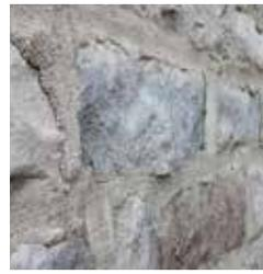
For a more old-world look, choose **overgrouting**. This technique uses a much heavier grout seam. Depending on the look you want, the grout can be even with or extend beyond the face of the stone, rather than being recessed like the standard grout technique. Grout may even partially cover the face of the stone. The overgrout technique is especially popular with larger, irregularly shaped stones.
