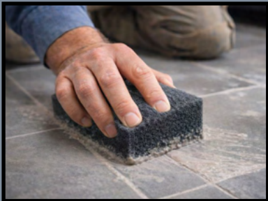
Emulsify epoxy or sanded grout
