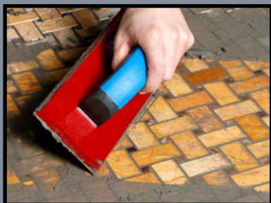
Urethane base cuts tight to the surface
