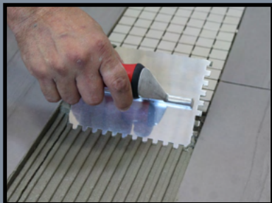
Perfect back splash & base-board trowel
