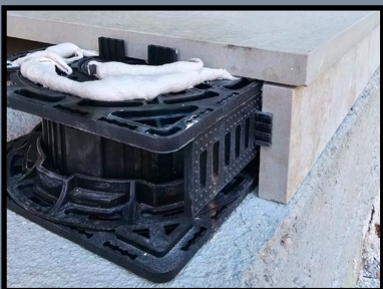
Facer plate is used for creating risers
