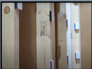
Install shims at 12" intervals on studs to achieve ultimate results
