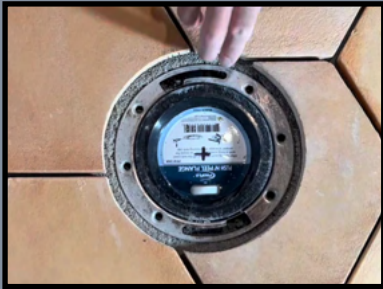
Perfectly center toilet flange holes in bathroom floor
