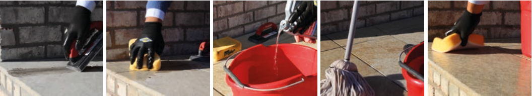
PIC 1. Fill joint with grout.
