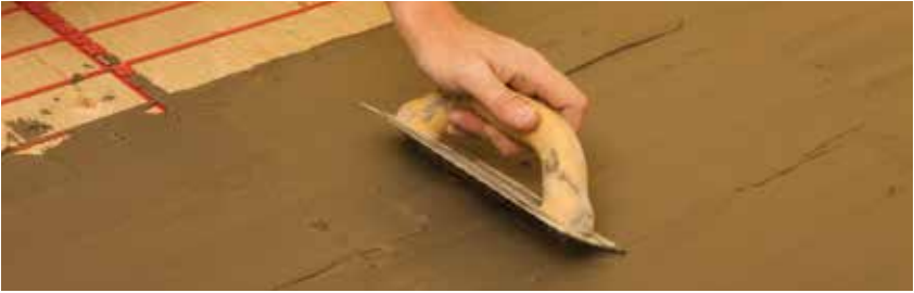
Figure 11: Mortar method
