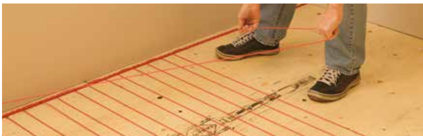
Figure 6: Install the heating cable
