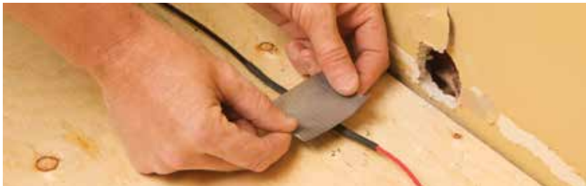
Figure 3: Secure the cold lead to the subfloor
