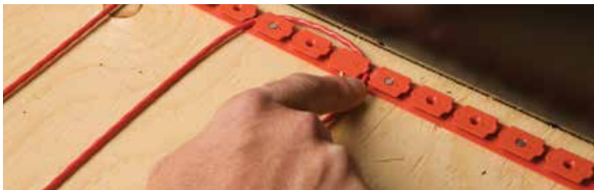
Figure 5: Install the heating cable
