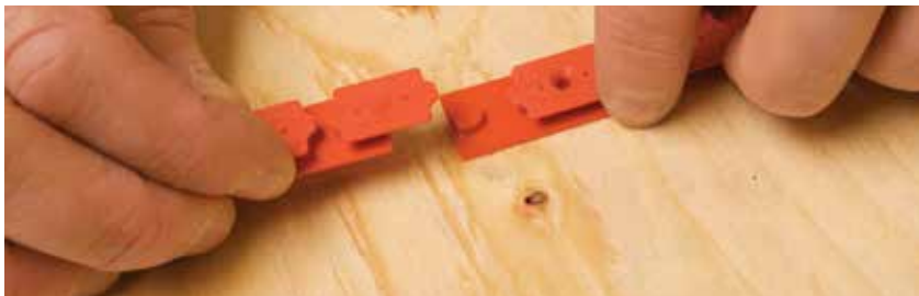
Figure 4: Snap together Mapeheat Cable Guides
