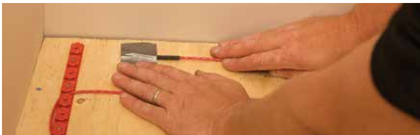
Figure 7: Secure the end seal
