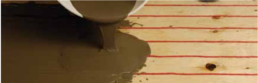
Figure 10: Self-leveling compound method
