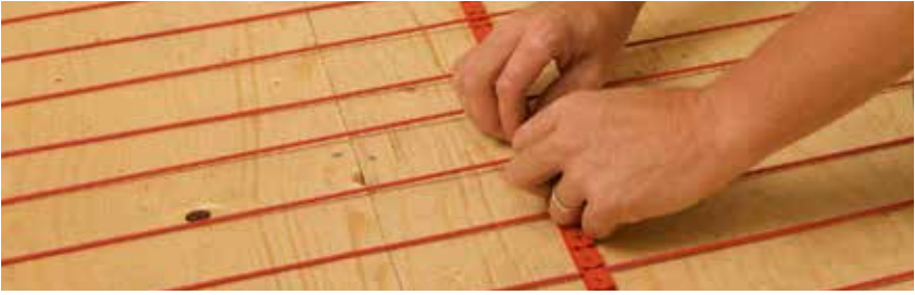
Figure 8: Install stabilizing guides
