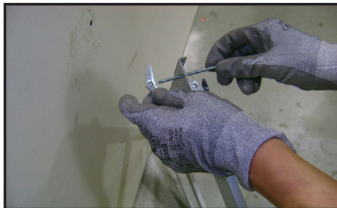
Figure 4.5 Toggle Bolt Installation through Mounting Bracket
