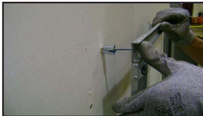
Figure 4.6 Installing Anchors in Hollow Wall
