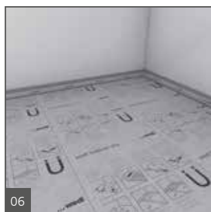
06 Use the Sealing Tape for the floor to wall junction. Apply the wedi 620 Sealant on the floor and a minimum and on the wall and lay the Sealing Tape into the wedi 620 Sealant.
