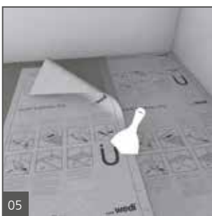
05 Spread flat all wedi 620 Sealant using a putty knife. Cross joints should be avoided.
