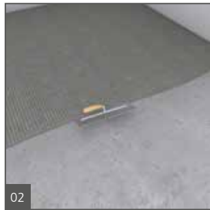
02 Apply Tile adhesive to the prepared subfloor using a 6 x 6 mm notch trowel.
