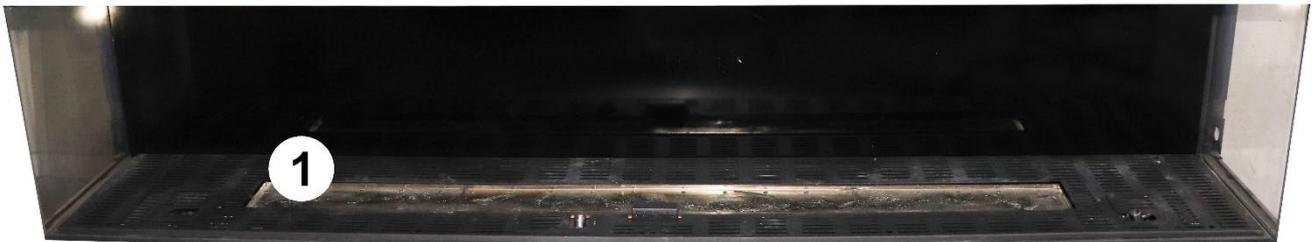
**⚠ WARNING:** For safety and optimal fireplace function, keep 1 inch around the pilot (behind pilot hood) completely clear of any media or debris.
