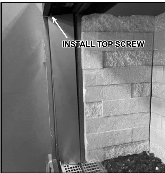
Figure 11.21 Transition Panel installed
