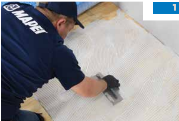
Apply thin-set to subfloor.
