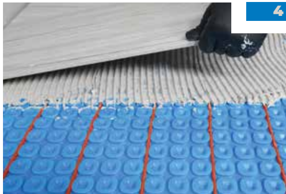
Trowel thin-set and install tile.
