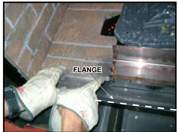
Figure 11.18 Positioning Left and Right Middle Base Refractory
