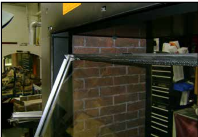
Figure 11.2 Initial Positioning of Frame into Opening.
