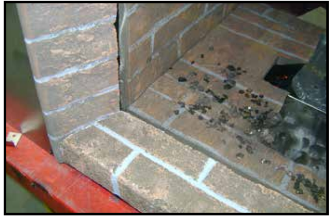
Figure 11.28 Outer Hearth Installation
