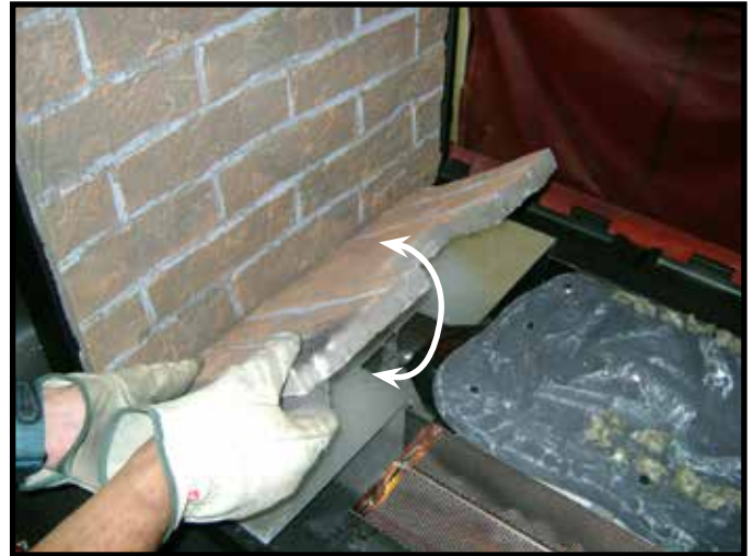
Figure 11.17 Positioning Inner Bottom Refractory
