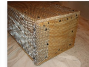
Building a new hearth out of plywood, followed by wire mesh, anchoring to floor, scratchcoat, then stone.
