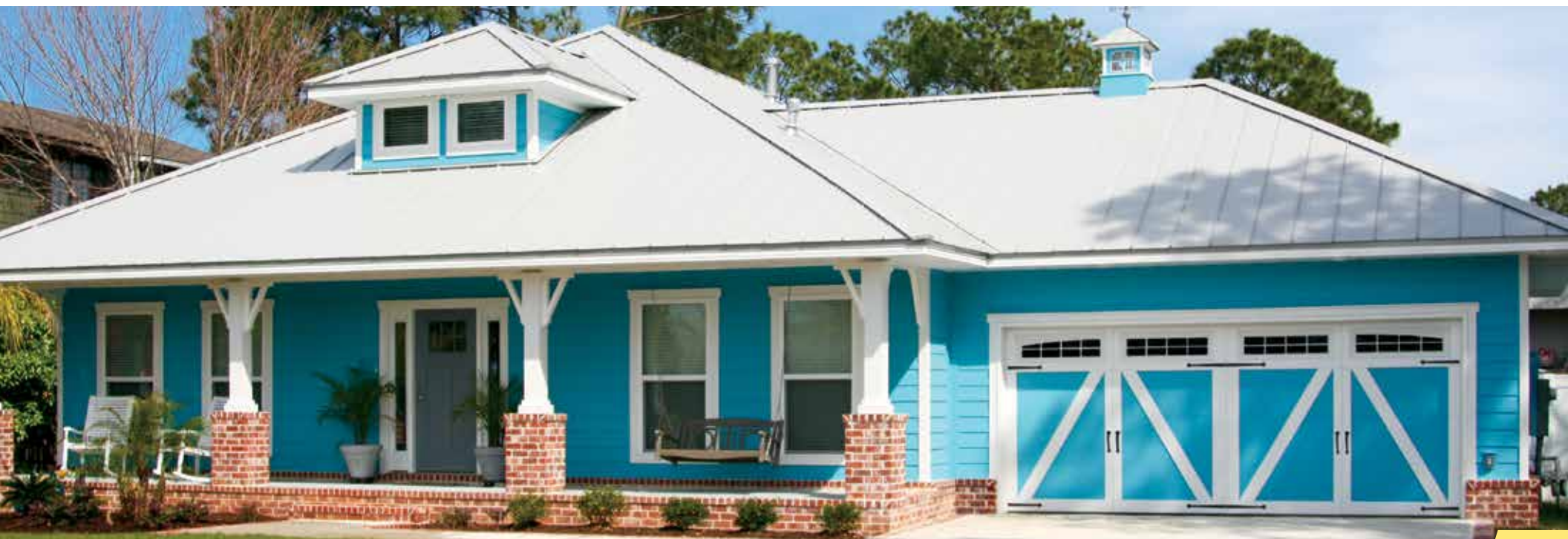
Model 8600, Springfield panel, Custom painted after installation, Arched Stockton windows
