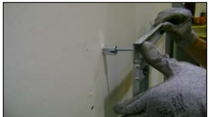
Figure 3 Installing Anchors in Hollow Wall
