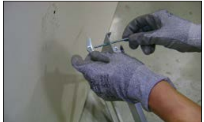
Figure 2 Toggle Bolt Installation through Mounting Bracket
