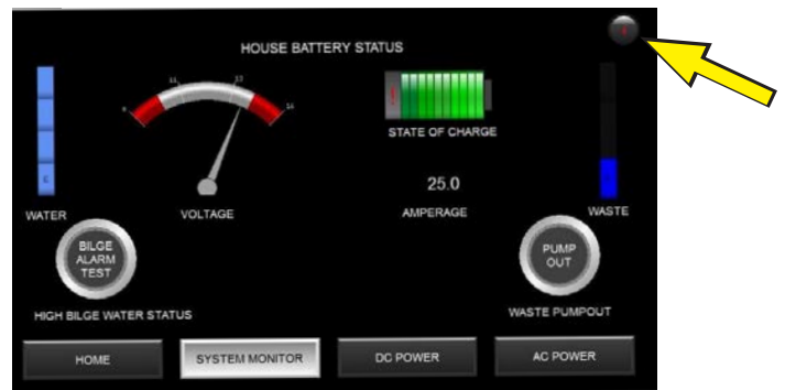
Power-up panel’s Home and System Monitor screens. Note the information icon in the upper right-hand corner.
