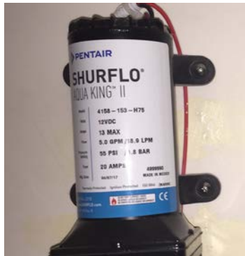
Fresh water pump, in the mechanical space
