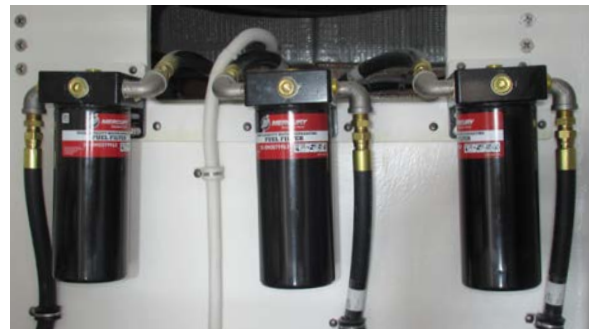
Gasoline fuel water separating filters (typical)
