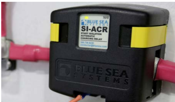
Automatic charging relay box (typical)
