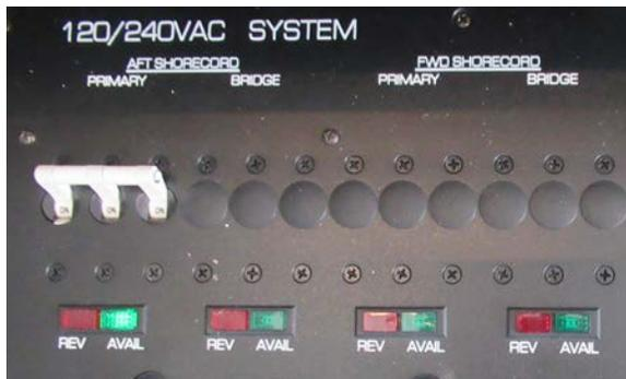
*Shore power and generator indicator lights, on the AC distribution panel*
