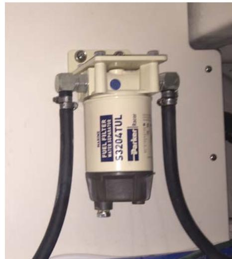
*Generator water-separator fuel filter*
