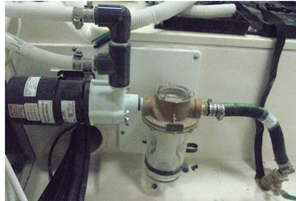
*Typical air conditioning pump, strainer, and valve, in the engine room*
