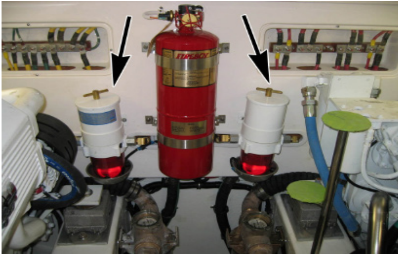
Figure 3-1: Centerline looking forward.
