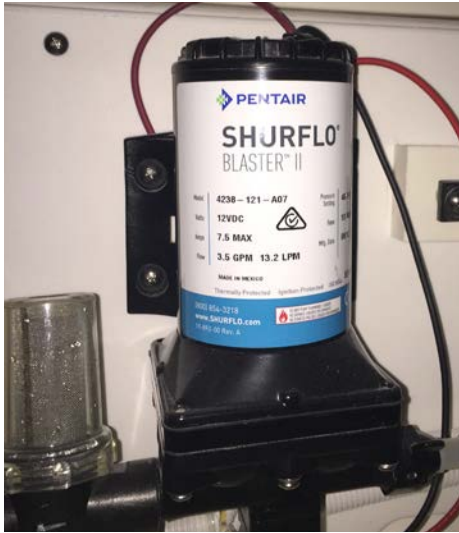
Typical raw water strainer (left) and pump
