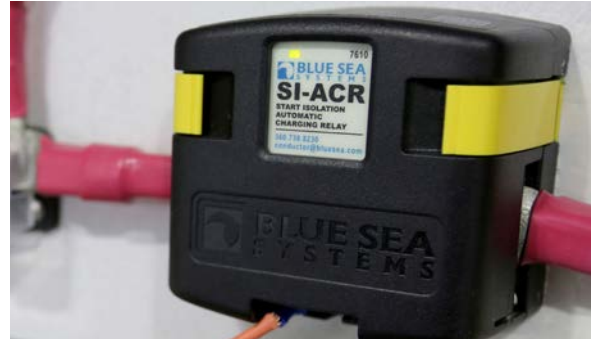
Automatic charging relay box (typical)
