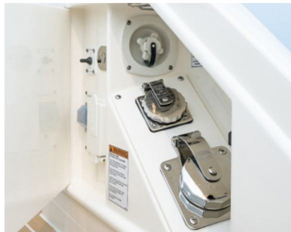
Aft shorepower cabinet
