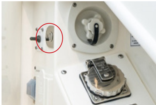
Engine flushing system start button (circled) in the aft shorepower locker
