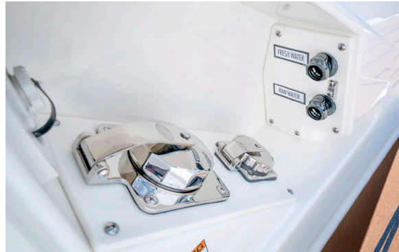
Shore power cabinet
