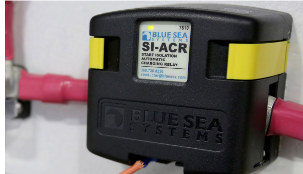
Automatic charging relay box (typical)
