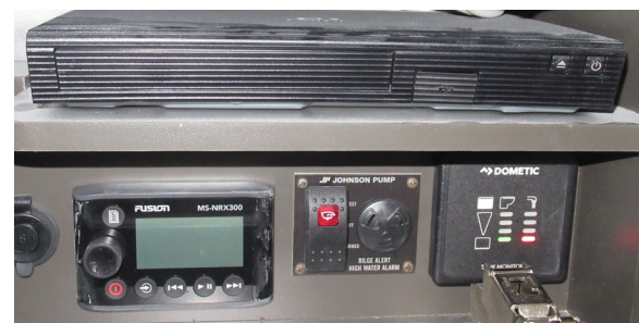
Cabin lower electrical cabinet
