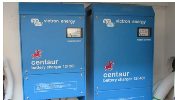
Battery chargers (typical)
