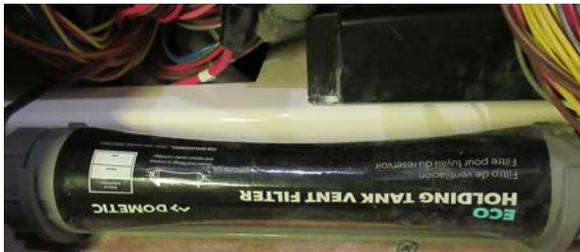
*Tank vent air filter, behind access panel in head compartment*
