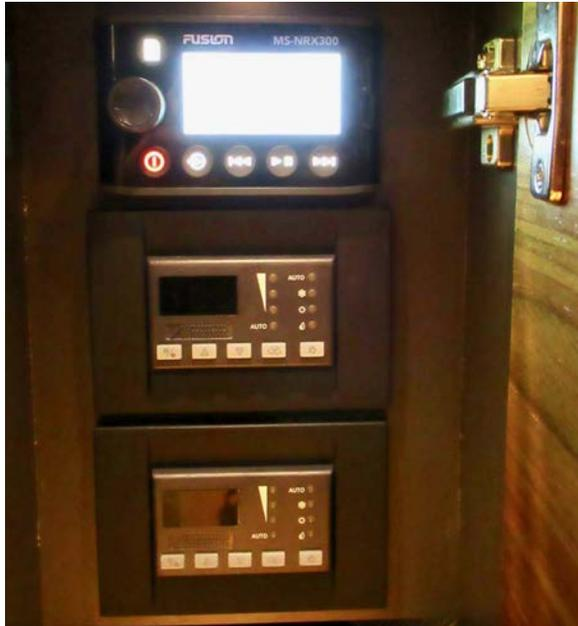
*Climate control panels and stereo remote control panel, located in the starboard berth cabinet*
