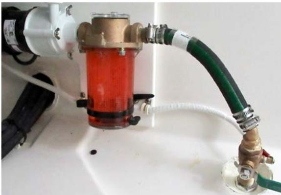
*Air conditioning pump, strainer, and valve*
