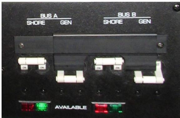
*Shore power and generator indicator lights, on the AC distribution panel*
