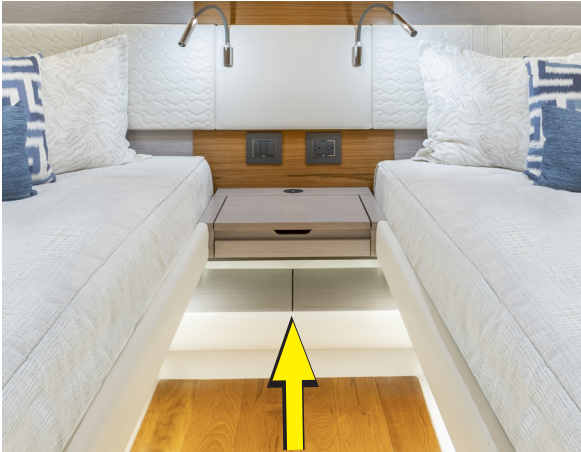
Pull the lower shelf up and out to access the shower sump and overboard discharge seacock
