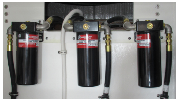
Gasoline fuel water separating filters (typical)
