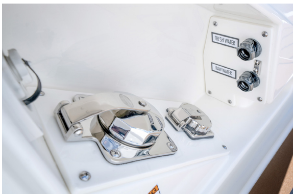
Aft starboard shorepower locker
