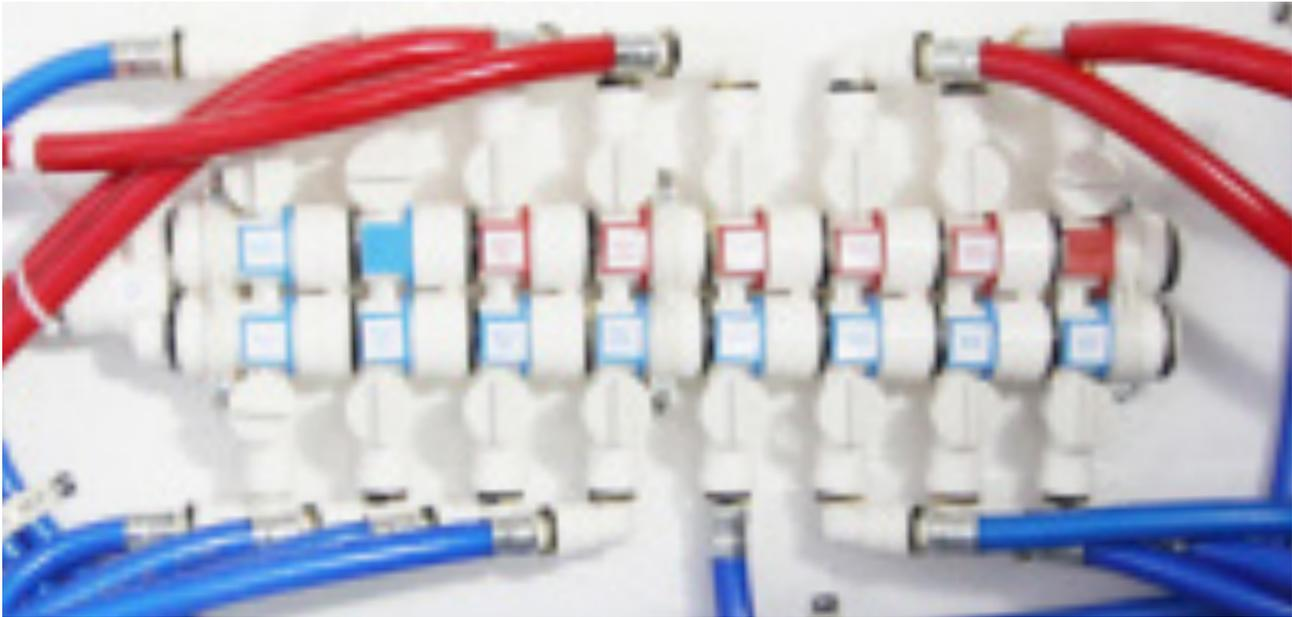
Figure 3-8: Fresh water system distribution manifold
