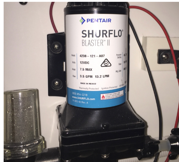
Typical raw water strainer (left) and pump
