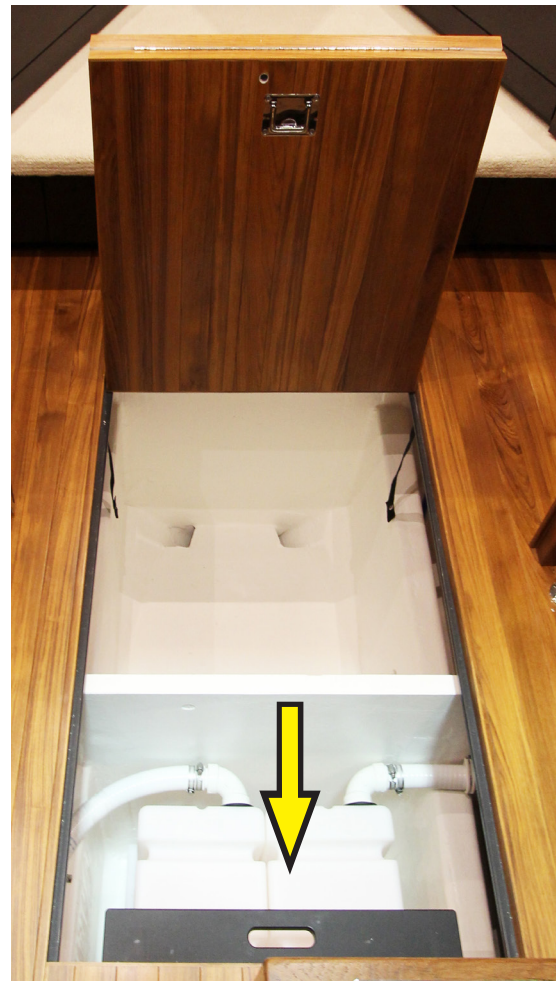
Figure 7-5: Atrium floor hatch and waste tank indicated by the arrow.
