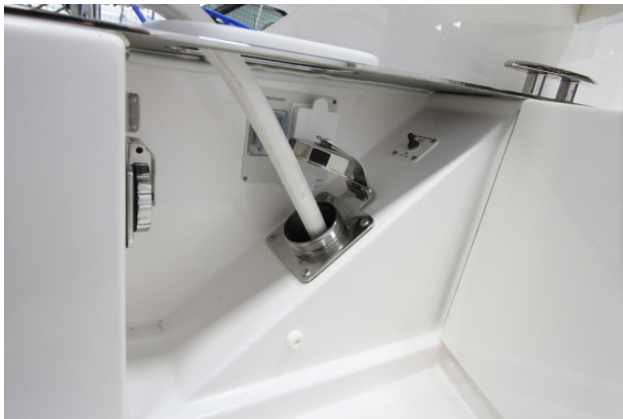
Figure 1-9: Aft shore power locker
