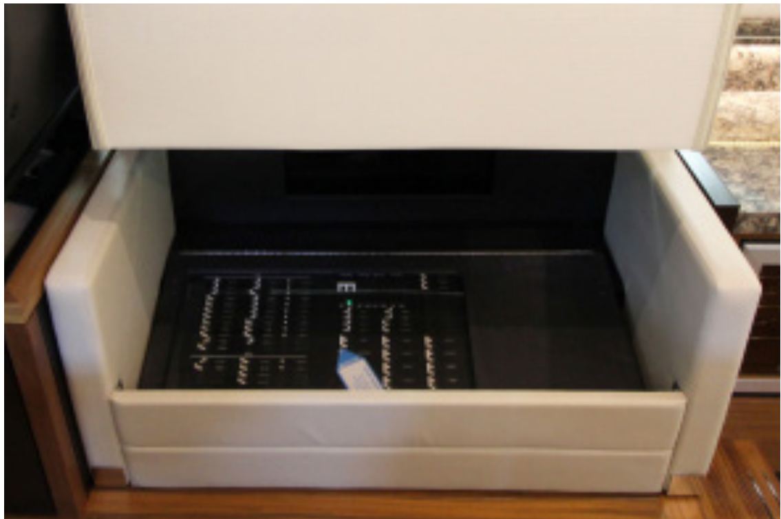
Figure 1-4: AC and DC Distribution Panels
