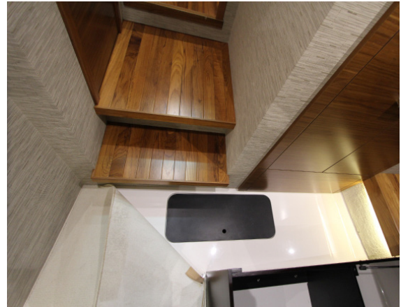
Figure 7-6: Overboard discharge seacock under master stateroom floor hatch
