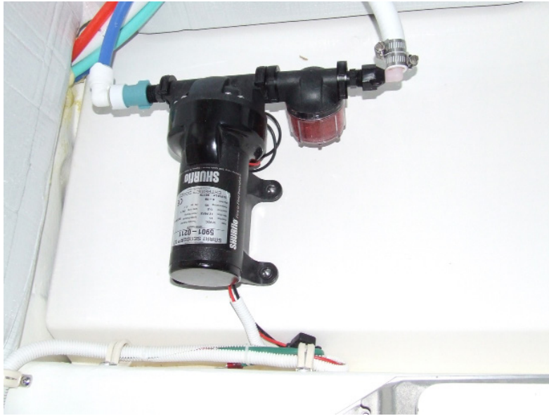
Figure 7-6: Fresh water filter and pump.
