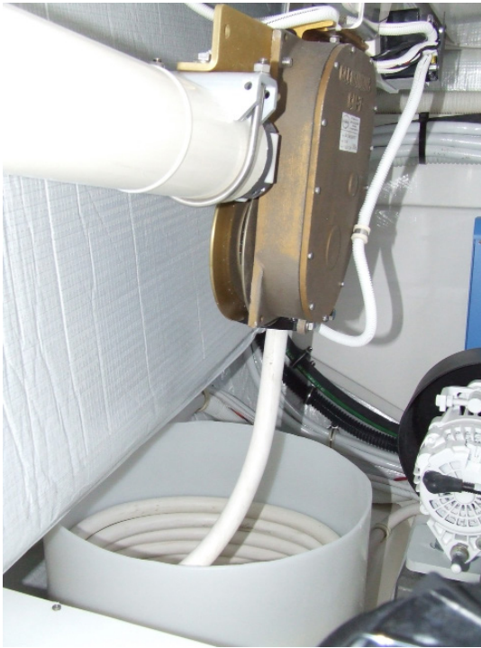
Figure 3-6: Storage bucket for the aft 50A, 240V shore power cable, outboard on port.
