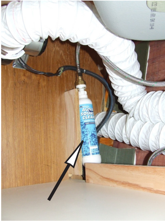
Figure 7-7: Access the galley inline freshwater filter under the galley sink.
