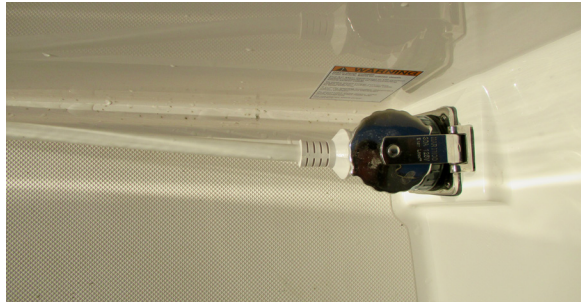
Shore power inlet, outboard of refrigerator
