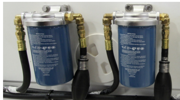
Gasoline fuel water separating filters (typical)
