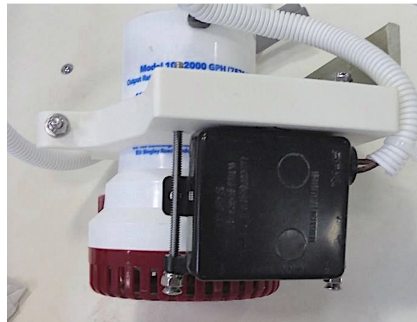
Typical bilge pump and float switch (right)
