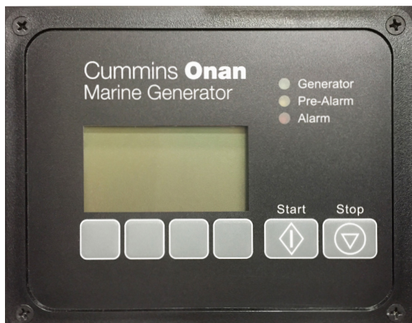
Remote generator control panel (typical)
