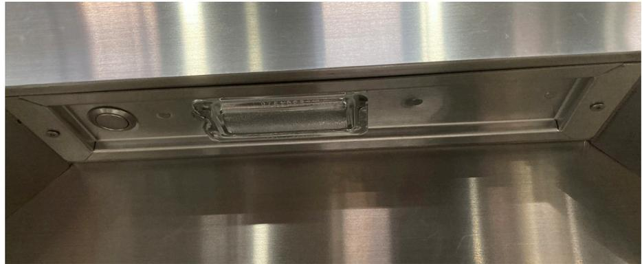
If the light does not work, check the bulb connections are tight (tiny screws on each side of the ceramic bulb holder), or replace the bulb itself with a new G4 "Bi-pin" 20W halogen bulb. You must loosen the screws to replace the bulb.
