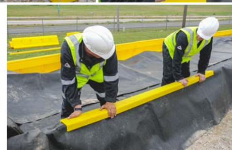
Large clips (included) hold the liner in place. Excess liner can be trimmed if desired.
