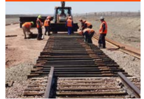
5 RAILROAD CONSTRUCTION FULL DESIGN/INSTALLATION SERVICES
