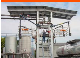
16 WEATHER PROTECTION LOADING SHEDS & CANOPIES
