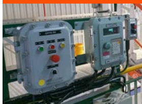
17 GROUNDING SYSTEM FOR TRUCK AND RAILCAR
