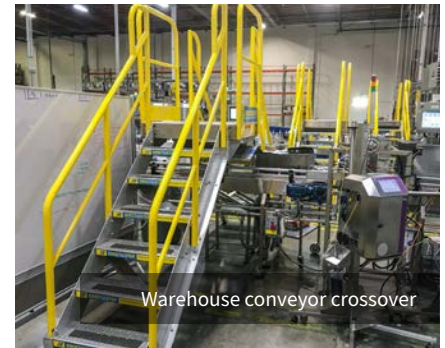
Distribution center machine access
