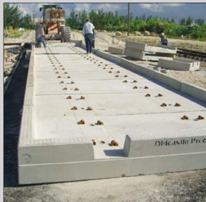
Railcar cement spill containment berm
