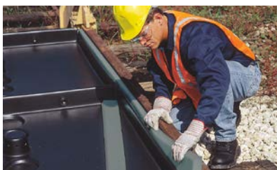
Closed-cell, polyethylene gaskets are then installed to provide a seal between the Pans and rails. (Black gaskets are provided.)
