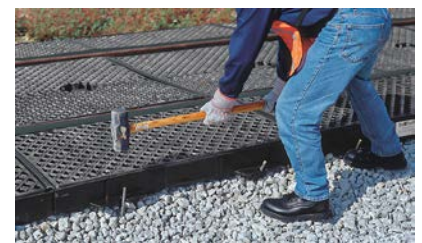
Side Pans are secured in place with 24" rebar fasteners. Typical installs require 2 pieces of rebar per Side Pan.
