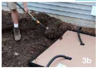
Below: A 4x4 basin is covered during backfill.
