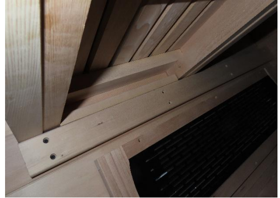
Wood Plank Between Underside of LOWER BENCH
