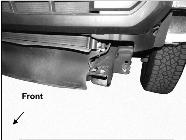
(Fig 5) Remove tow hooks (driver/left side of frame pictured)
