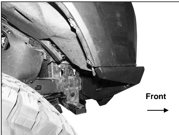
(Fig 19) Passenger/right side of bumper cover and flare cut to fit Hilne Wing
