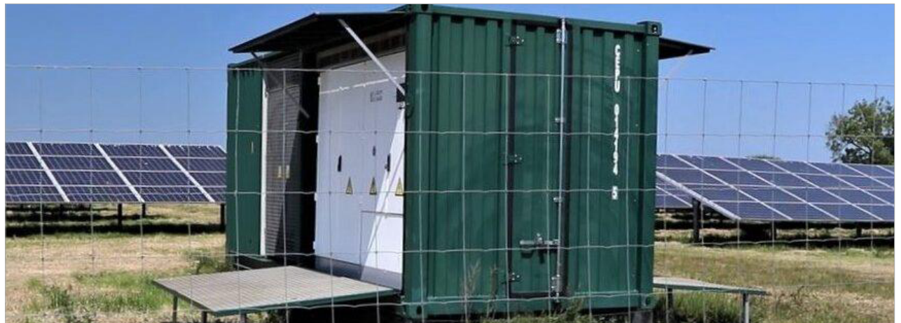
PHOTO: A typical field inverter station
