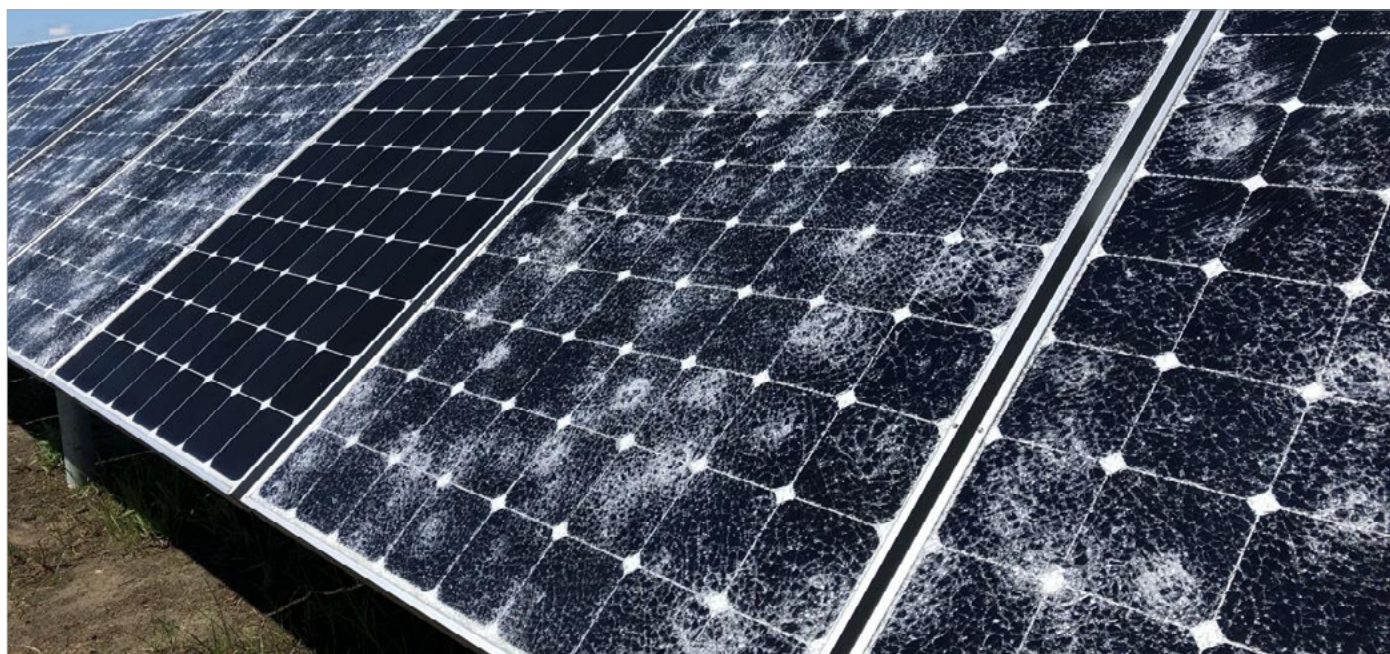
Fig 01 – Hail damage to solar panels
