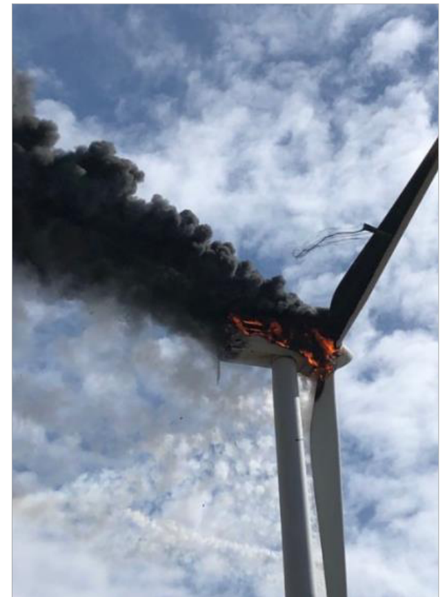
FIG 07 - Nacelle fire in wind turbine
