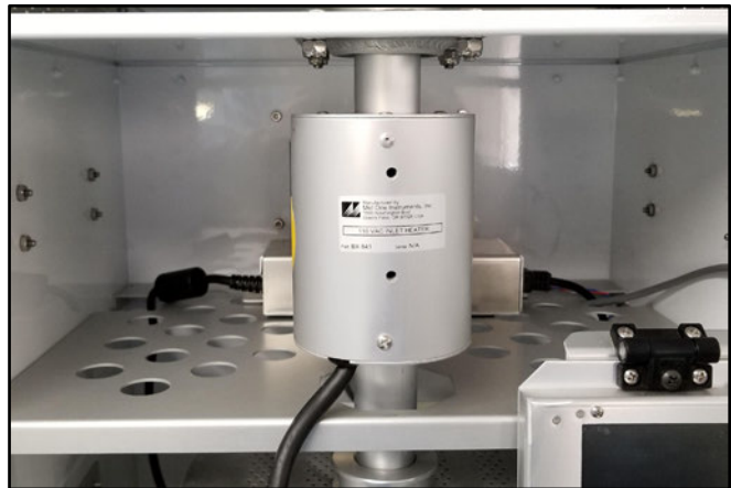
Figure 4-10 Inlet and Heater Installed
