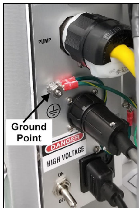
Figure 4-17 Ground Cable Installed
