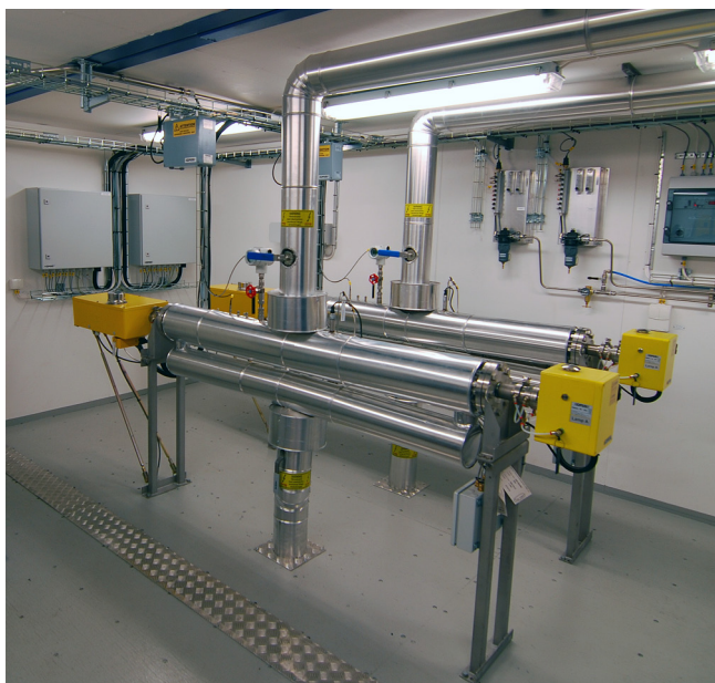
A fast loop installation
