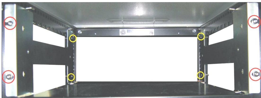
Figure 29 Installation of rack mount brackets
