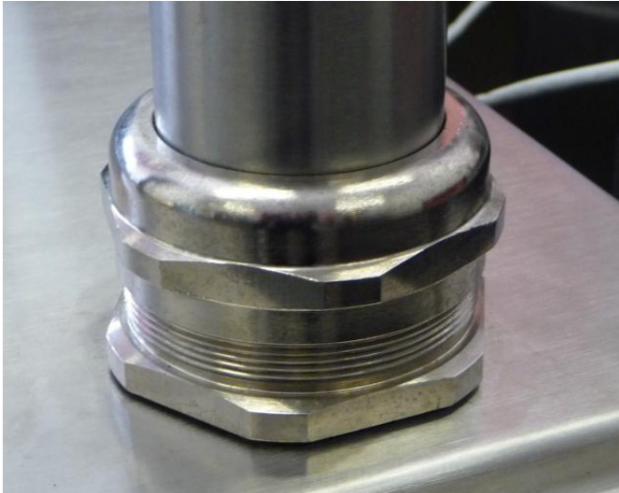
Fig. 8: Fixing of the weather station tube
