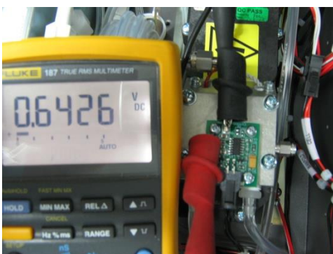
Figure 57 – Typical Test Point Reading of Internal Pump Pressure Sensor
