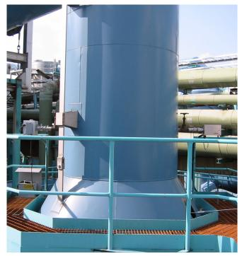
A cross-stack installation, showing the emitter and receiver
