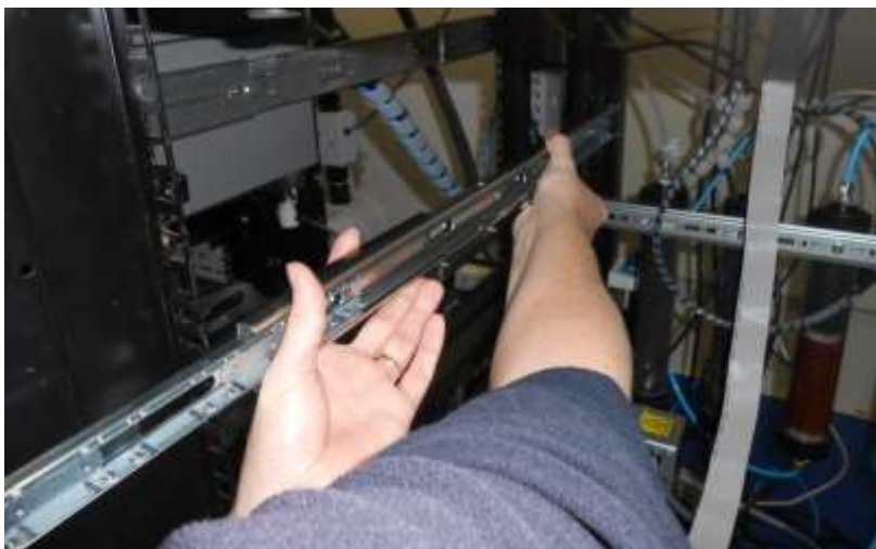
Figure 101 – Test Fit the Rack Slide Assembly into your Rack
